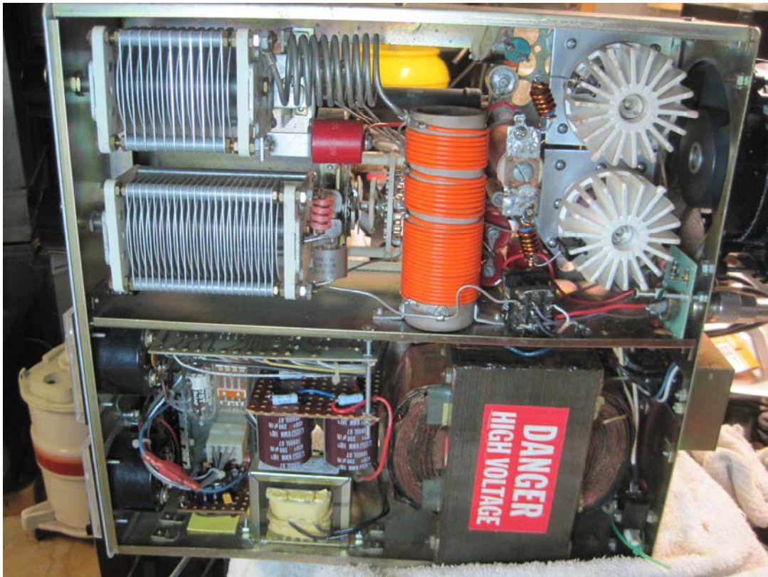
Completed Conversion – Top View
